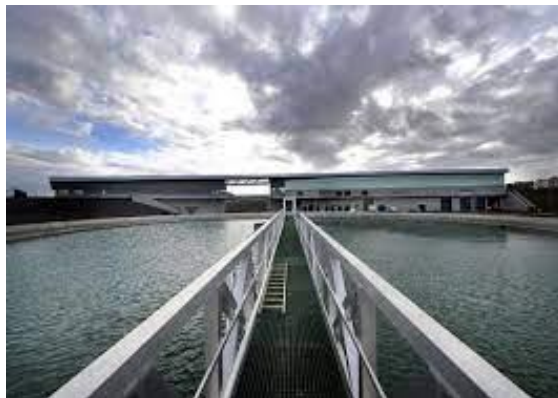
Figure 13 - Station d'épuration - Mainvilliers
